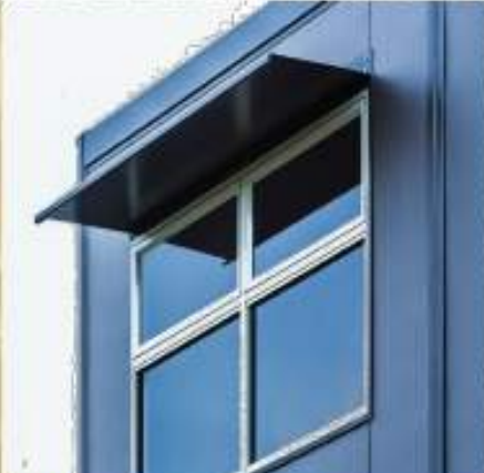
Solar Hoods Paint Dulux Marais GR 13
