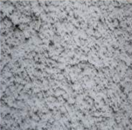
Walling and Slab Edges
